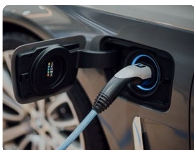
EV chargers in secure parking
